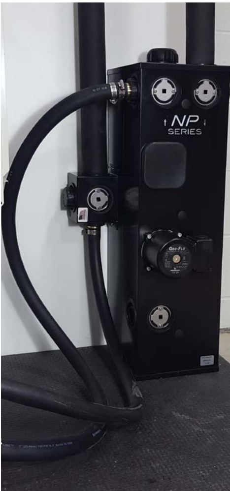
Figure 7: Flow center mounted 3-way valve
