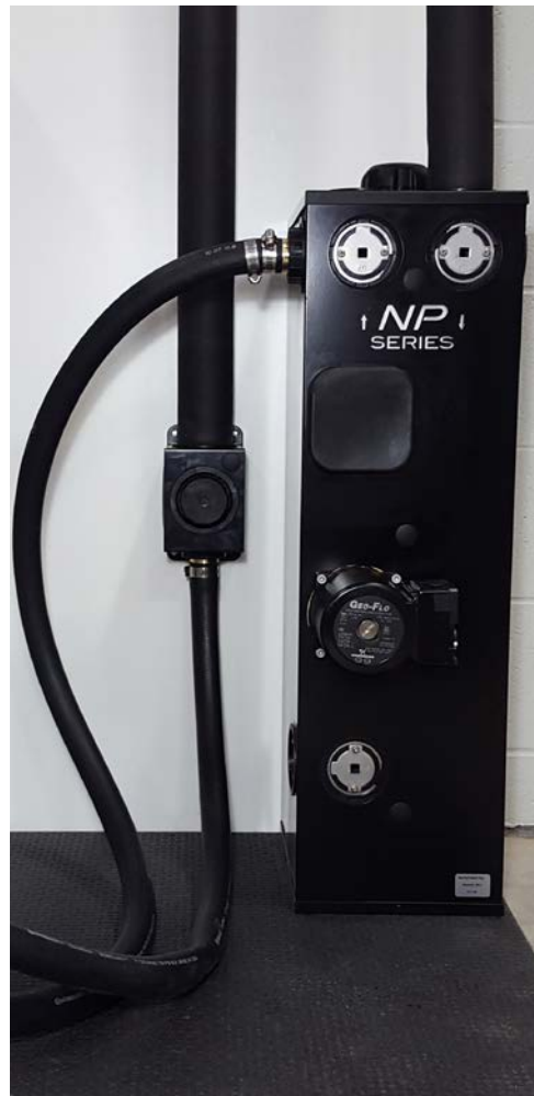
Figure 8: Wall mounted 3-way valve
